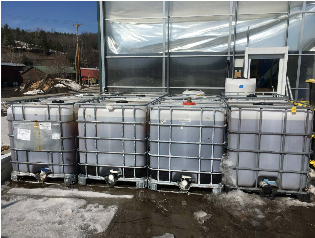
IBC totes filled with urine. Note melting snow in foreground—these tanks store frozen urine throughout the winter without damage.
