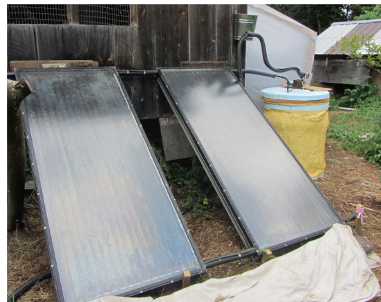
Solar pasteurizer: solar panels on left, insulated urine tank behind on right.
