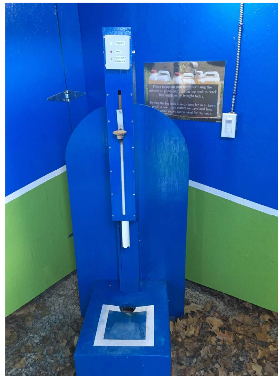
Self-service vacuum pump-out station for emptying 5-gallon jugs of urine at the collection depot.
