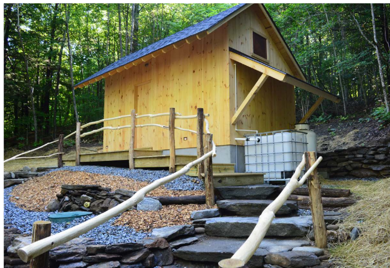
Urine collection tank connected to a urine-only toilet at a summer camp for girls in Vermont.
