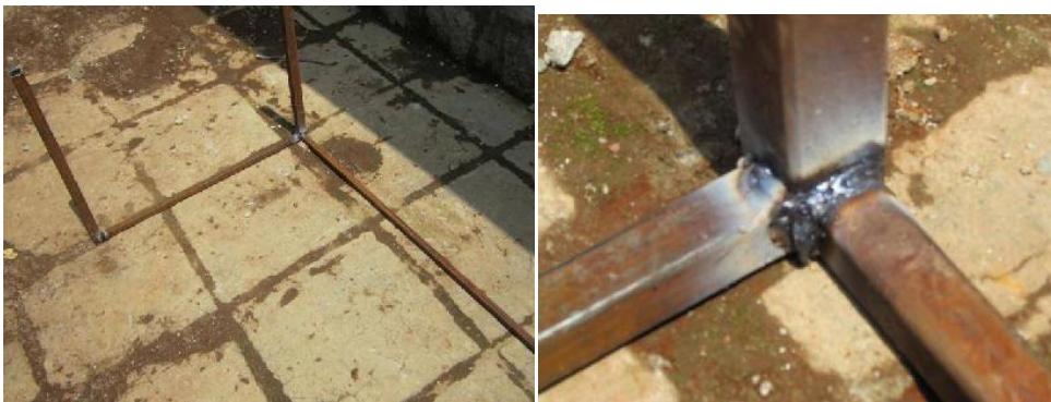
Picture 2: Image of 120.5cm square pipe connection (left) and flush connection at corner (right)
