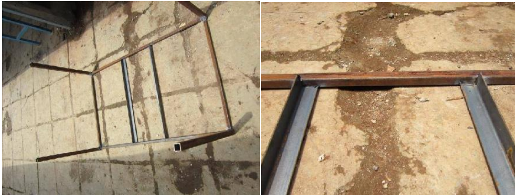
Picture 6: Image of first (left) and second (right) angle bar placement
