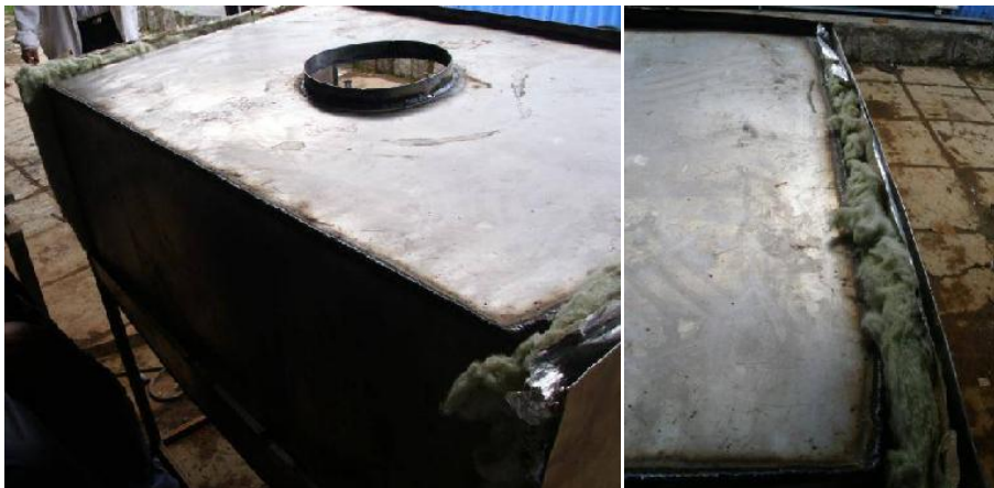
Picture 62: Image of fiberglass sides inserted (left) and close up of side with fiberglass inserted
