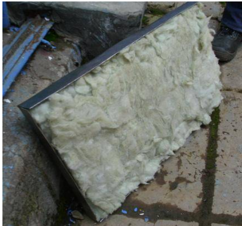
Picture 41: Image of insulation added
