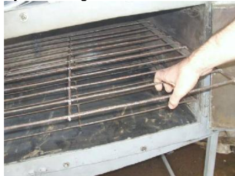
Picture 88: Image of rack removal
