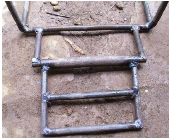
Picture 76: Image of interior bars added
