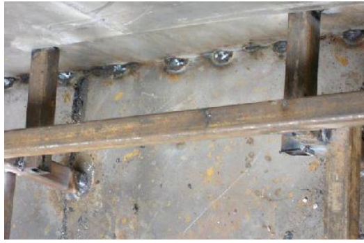
Picture 57: Close-up view of supports
