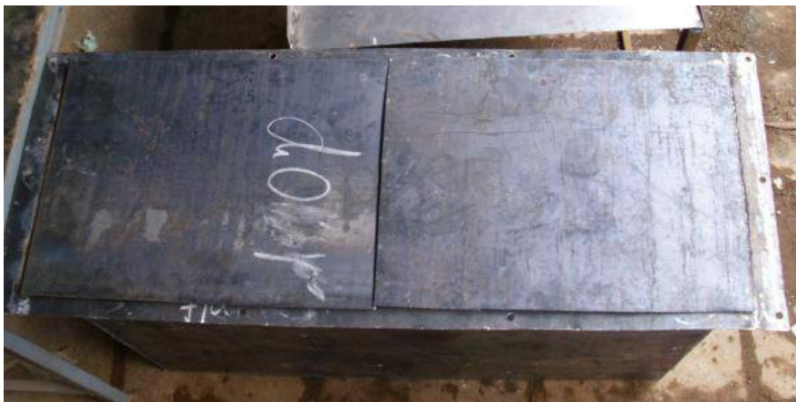
Picture 43: Doors in combustion chamber
