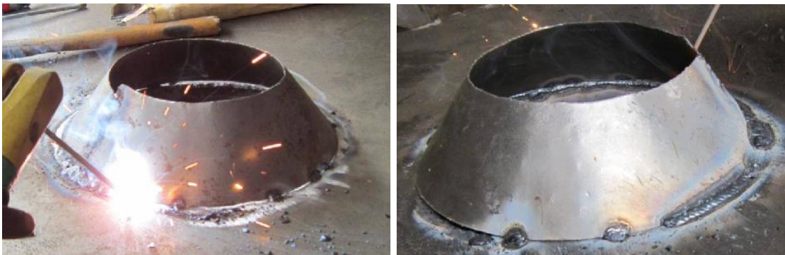
Picture 68: Images of the welding for a hermetic seal
