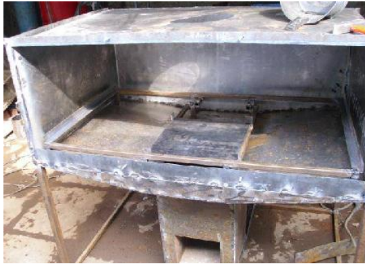
Picture 59: Image of side/top piece attached
