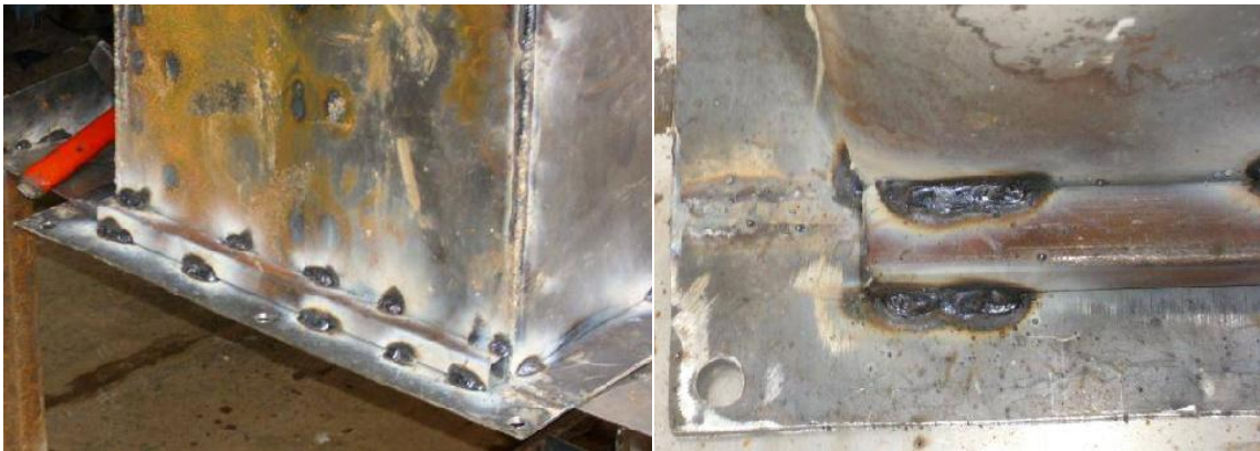
Picture 37: Square pipe attached to the back of the baking chamber flange (left), flush with top and bottom (right)
